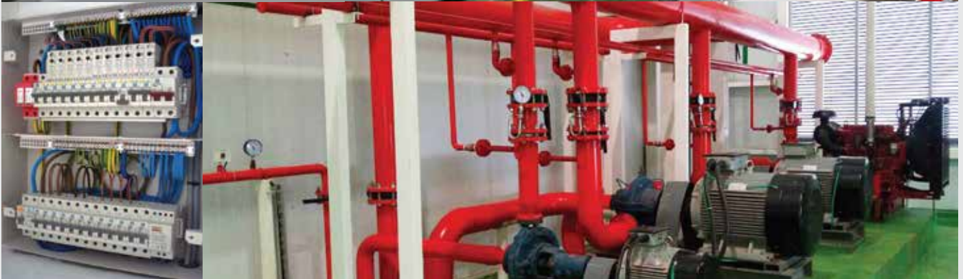
Turnkey Project : Electromechanical, MEP, HVAC and Fire fighting sytem
