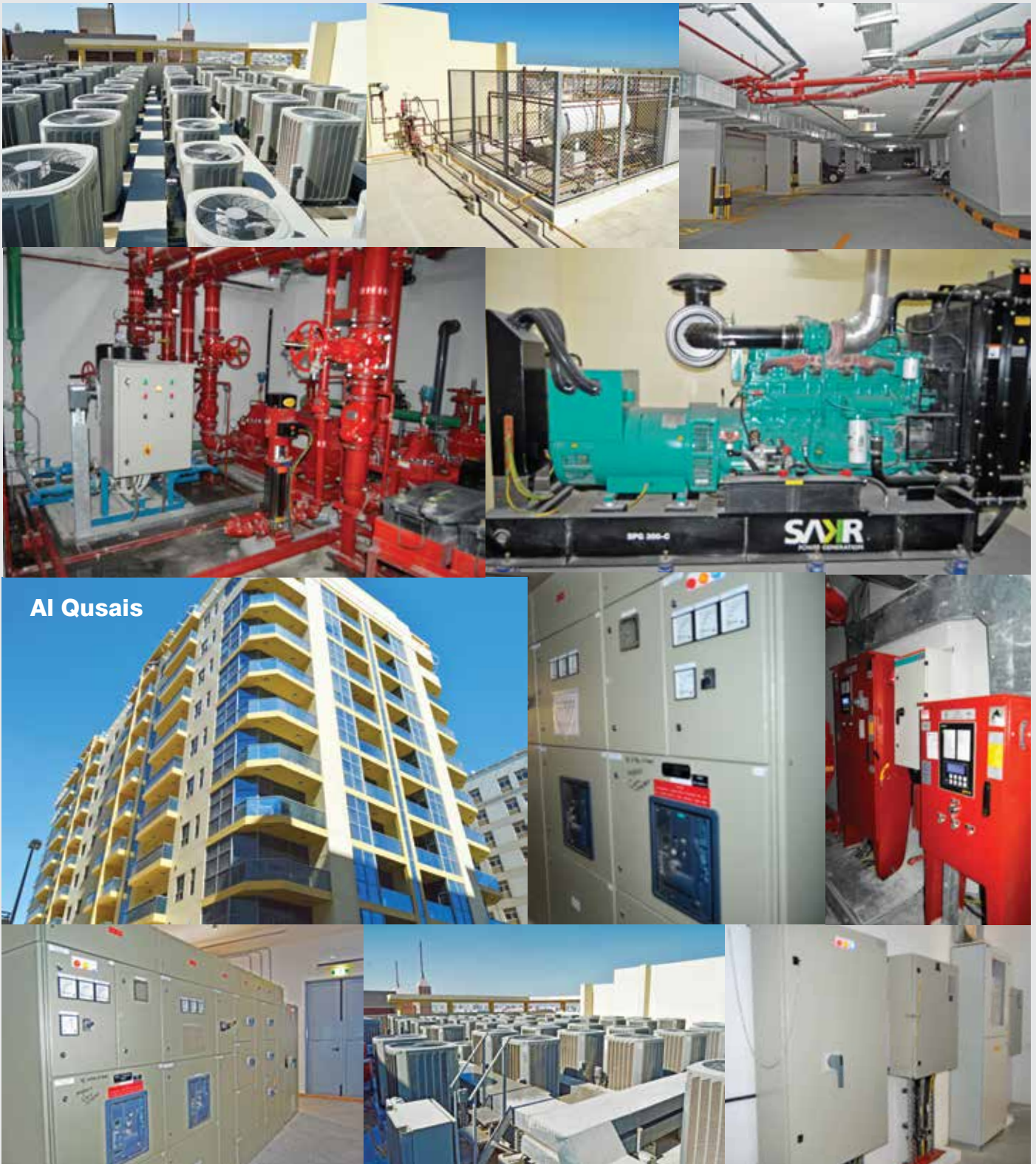
Turnkey Project : Electromechanical, MEP, HVAC and Fire fighting system
