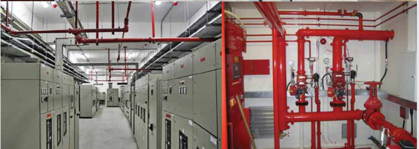
Turnkey Project : Electromechanical, MEP, HVAC and Fire fighting sytem
